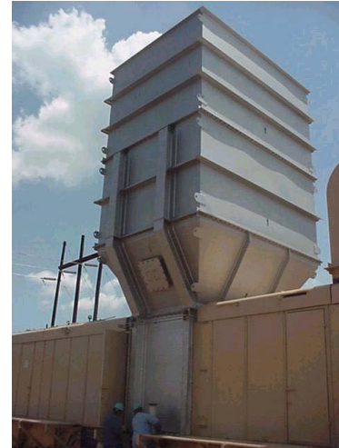
GE Frame 5 Inlet Silencer and Ductwork and Exhaust Silencer and Stack
