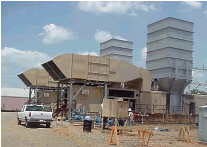
GE Frame 5 Inlet Silencer and Ductwork and Exhaust Silencer and Stack
