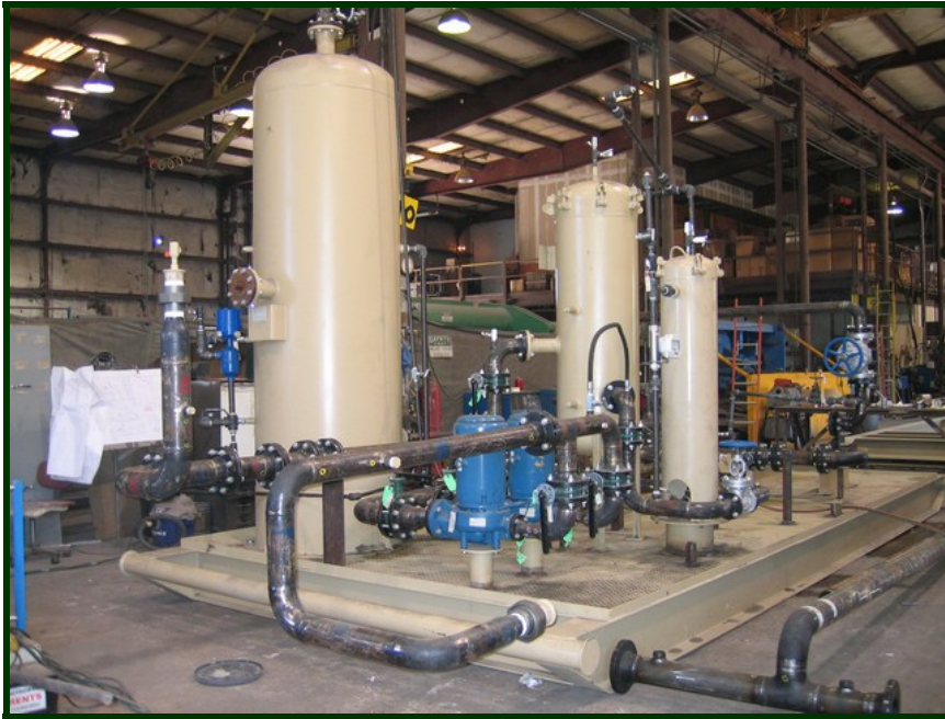
Regeneration Skid in fabrication
