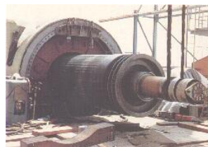
Generator Turbine Removal
