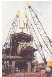
GE Frame 5 Turbine and Compressor Removal
