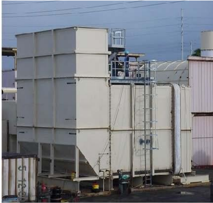
GE Frame 7 Exhaust Silencer and Ductwork
