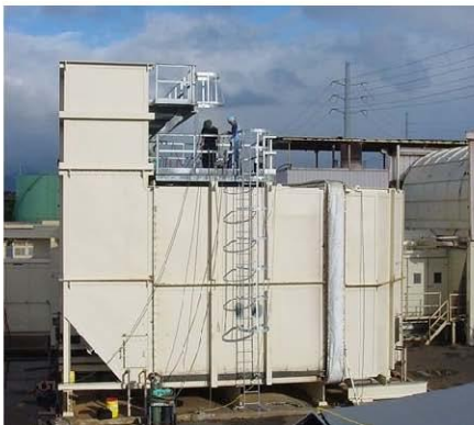
GE Frame 7 Exhaust Silencer and Ductwork
