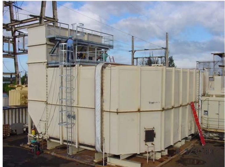
GE Frame 7 Exhaust Silencer and Stack
