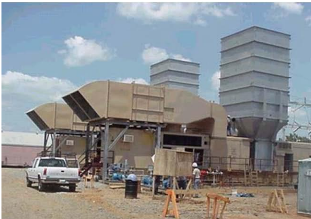
GE Frame 5 Inlet Silencer and Ductwork
