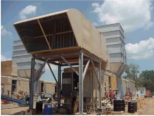
GE Frame 5 Inlet Silencer and Ductwork
