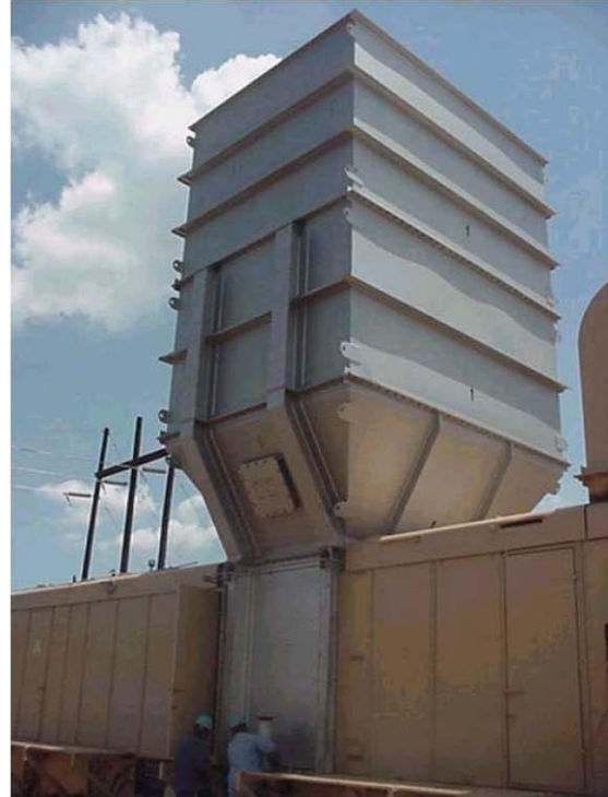
GE Frame 5 Exhaust Silencer and Stack
